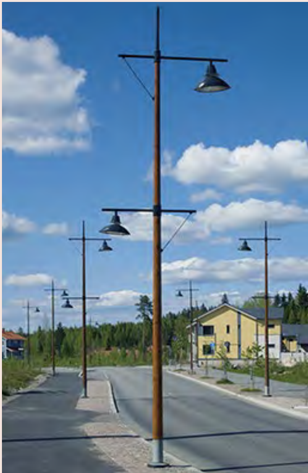
Wooden pole street lamp
