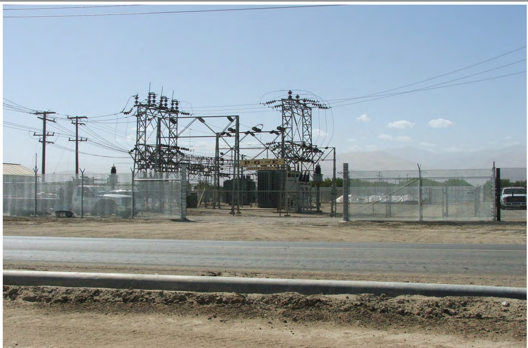
Existing PG&E Lakeview Substation
