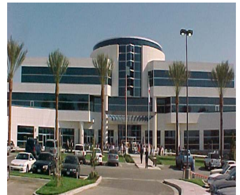
Public Facility Construction
